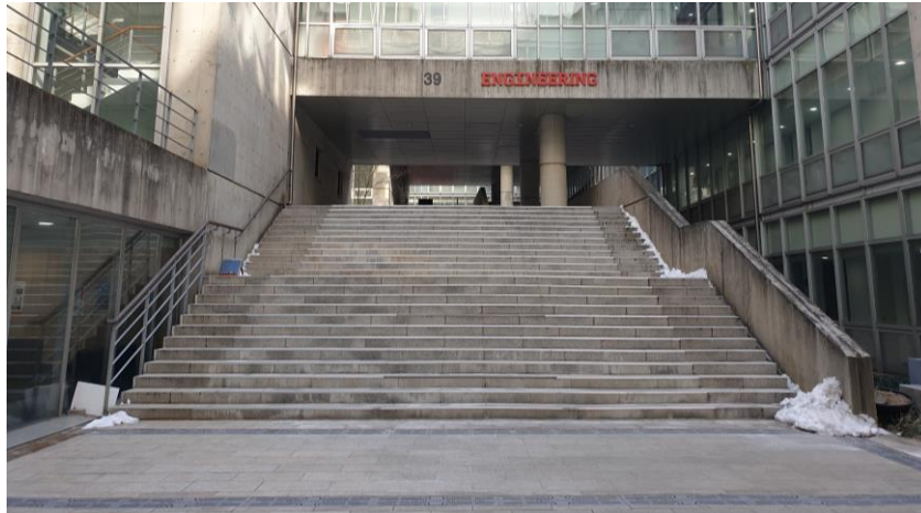
Front stair Bldg.39
