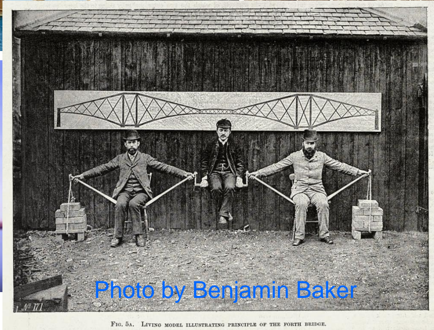
FIG. 5a. LIVING MODEL ILLUSTRATING PRINCIPLE OF THE FORTH BRIDGE.
