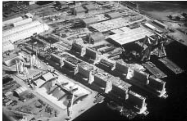
Figure 23 West Bridge, Prefabrication Yard
