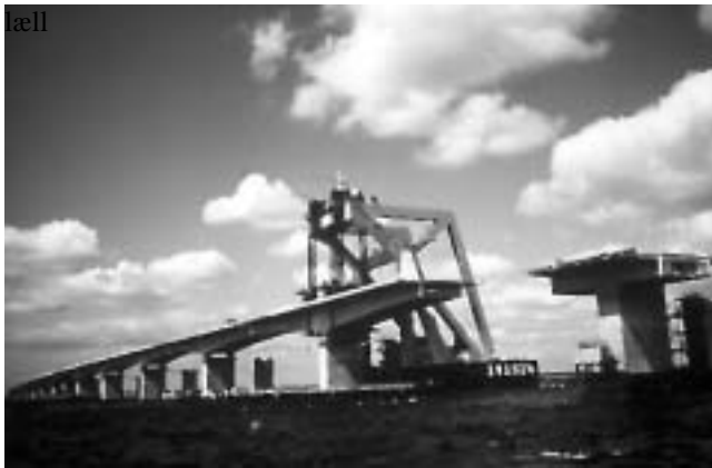
Figure 24 Erection of the Great Belt, West Bridge
