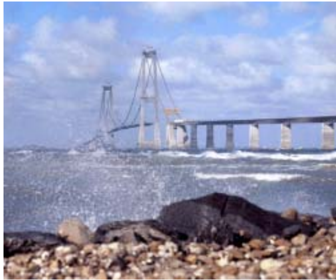
Figure 25 The Great Belt, East Bridge
