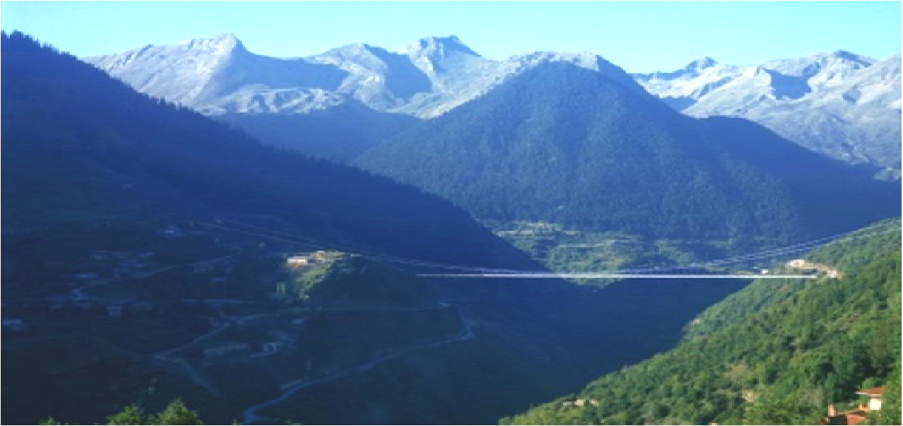
Fig. 21 The Metsovitikos Bridge Project in Greece
