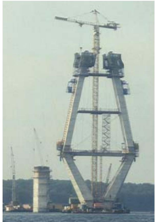
Fig.20 Pylon of the Farø Bridge under construction
