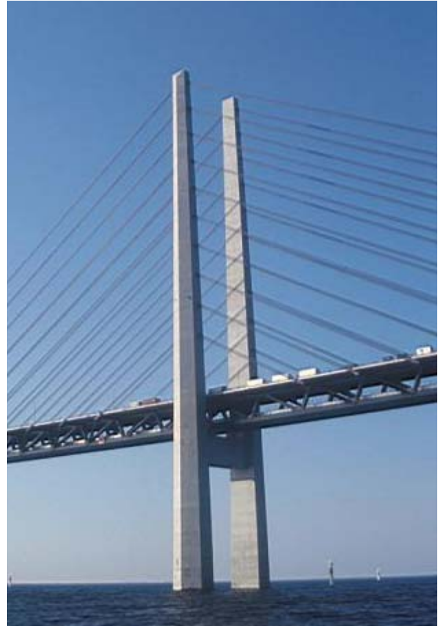
Fig.14 Pylons of the Øresund Bridge
