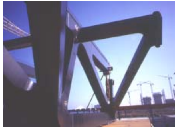
Fig.16 Outriggers of the Øresund Bridge
