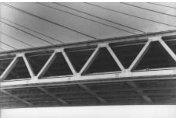
Fig.3 Double deck truss (Higashi Kobe Br.)
