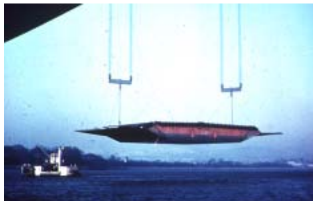
Fig.4 Streamlined box girder (Severn Br.)
