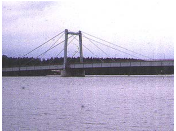
Fig.10 Pylon of the Strömsund Bridge
