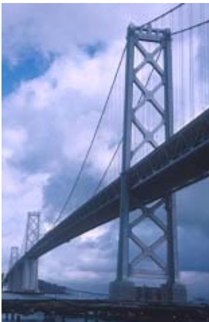
Fig.8 Pylons with diagonal bracings (Bay Bridge)
