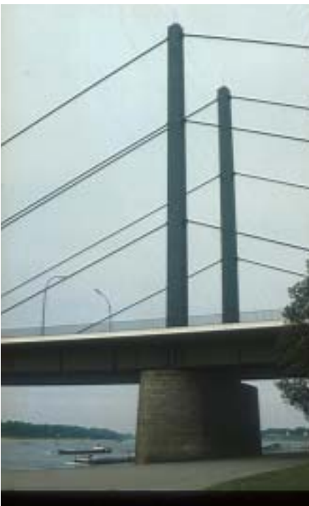
Fig.11 Pylon of the Theodor Heuss Bridge
