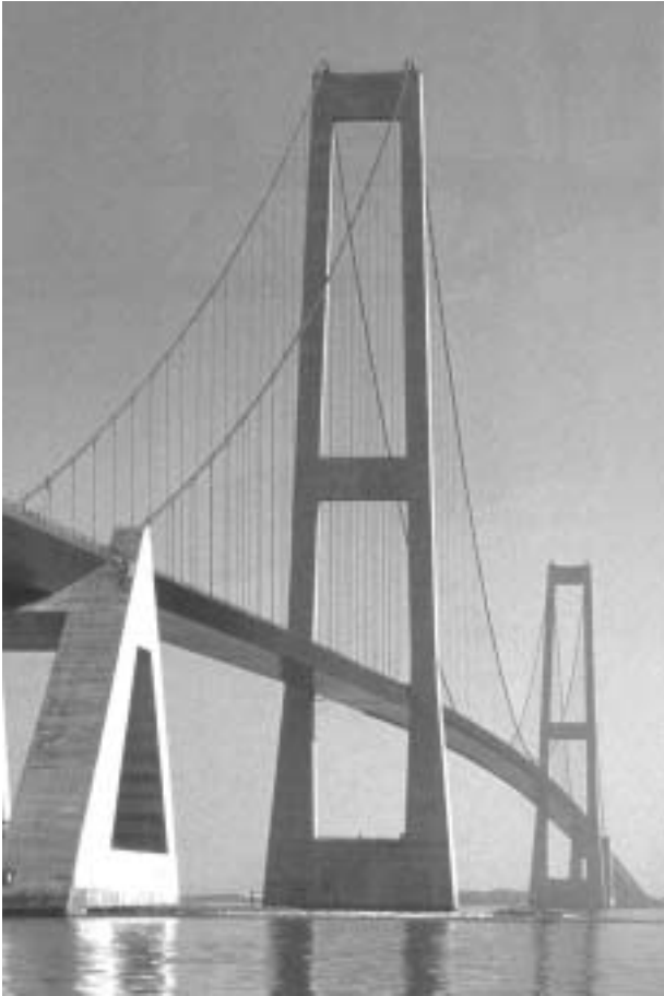
Fig.13 Pylons of the East Bridge
