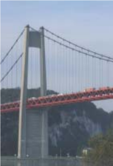
Fig.9 Pylon of the Tancarville Bridge
