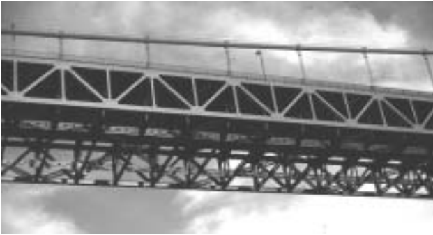
Fig.1 Stiffening truss (Golden Gate Bridge)
