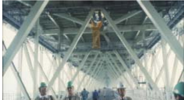
Fig.2 Cross bracings (Akashi Kaikyo Bridge)
