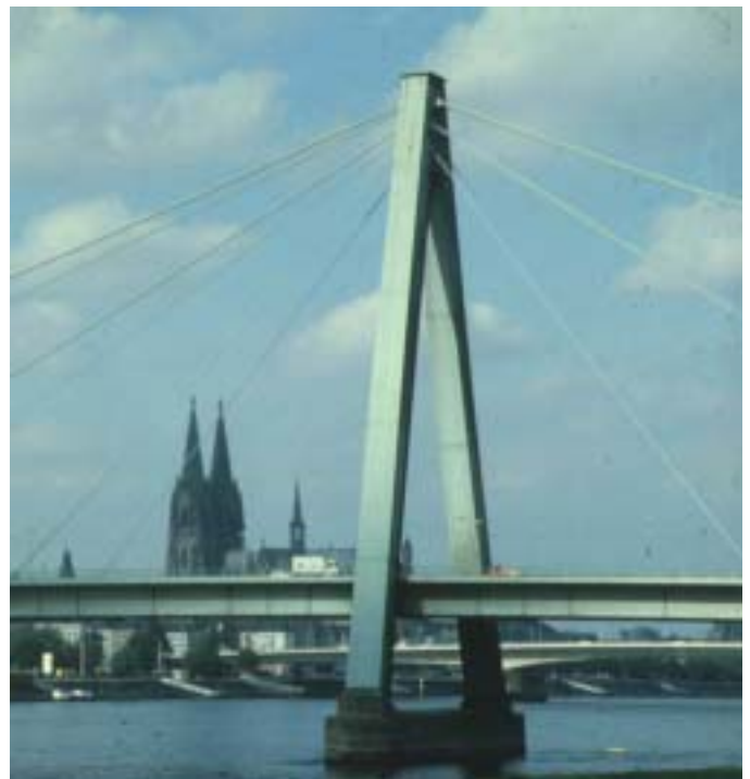
Fig.12 Pylon of the Severins Bridge
