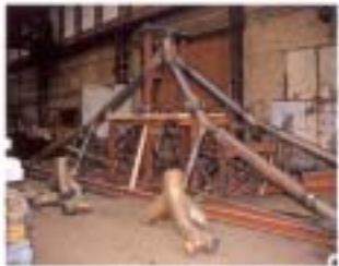
Pre-assembly of a tree-column from tubes with cast steel joints
